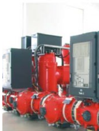
Gas insulated switchgear (GIS).
