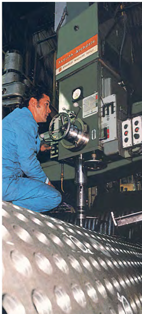
Steam drum drilling
