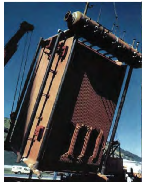
Eckrohrkessel corner tube boiler
