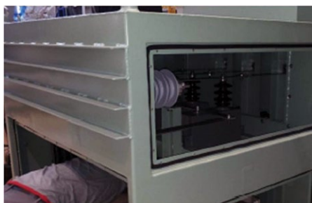
Voltage Transformer
