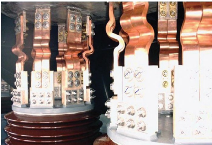
Copper flexible connections
