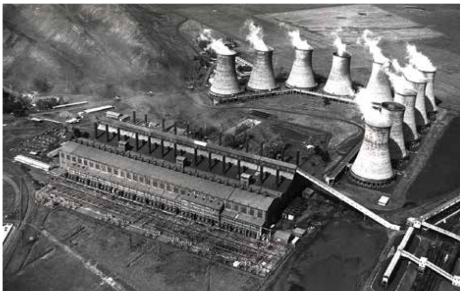
At 424 MW, mighty Klip was the largest power station in the Southern Hemisphere in 1939 and a magnificent showpiece of pre-war engineering expertise.
