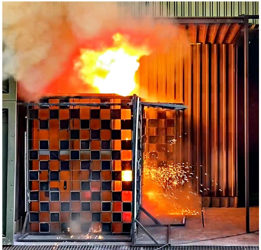
SBV4XE switchgear assembly undergoing an internal arc test at SABS NETFA.
