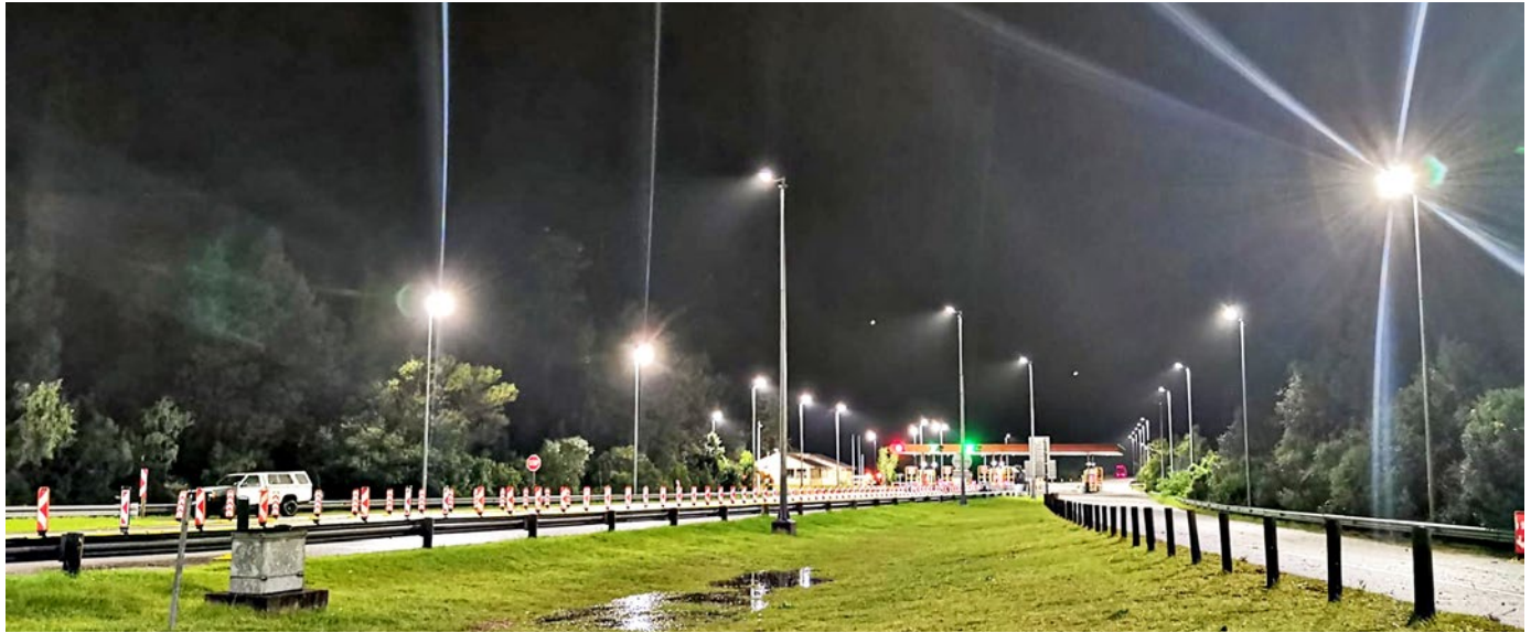
The Tsitsikamma Toll Plaza with Genlux's LED lights in place.
