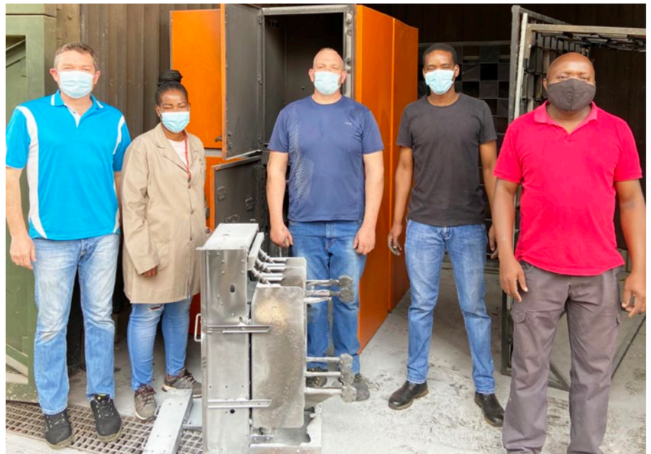
Posing in front of the SBV4XE panel assembly after a successful internal arc test at SABS NETFA are (from left): Rhett Kelly, MV Switchgear's Design & Development Manager; Millcent Chokoe, Senior Test Officer, SABS NETFA Short-Circuit Laboratory; Piet Ferreira, MV Switchgear's Engineering Manager; Zinhle Nkosi, MV Switchgear's Development Assistant; and Seth Mnisi, Manager, SABS NETFA Short-Circuit Laboratory.
