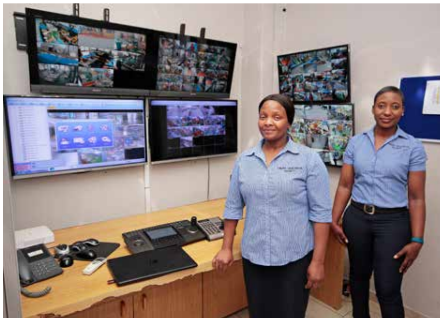
From left to right – Dorcas Nkomo and Nokuzola Majebe, the owners of Thembaukukhanya Security in their CCTV monitoring control room.
