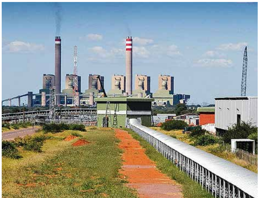
A view of Medupi power station near Lephalale, Limpopo Province (Photo sourced from Mining Weekly).
