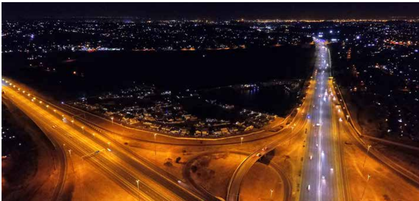
This picture shows the R21/N14 interchange in Pretoria with the N14 extending northwards where the GEN 2 LED streetlights, manufactured and supplied by Genlux Lighting, have been installed. The white LED lights contrast against the yellow High Pressure Sodium (HPS) HID lights in the foreground.
