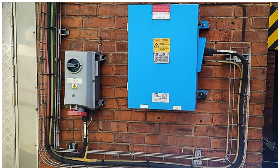
A view of one of the first DC chop-over boxes developed and manufactured by Static Power to facilitate the prompt and safe provision of temporary power to substations.
