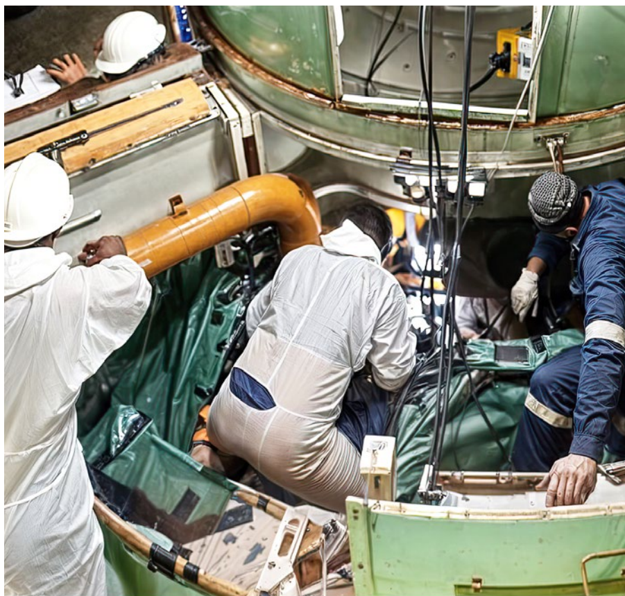
The Voith team machining the rotor rim at Steenbras Hydro Pump Station.
